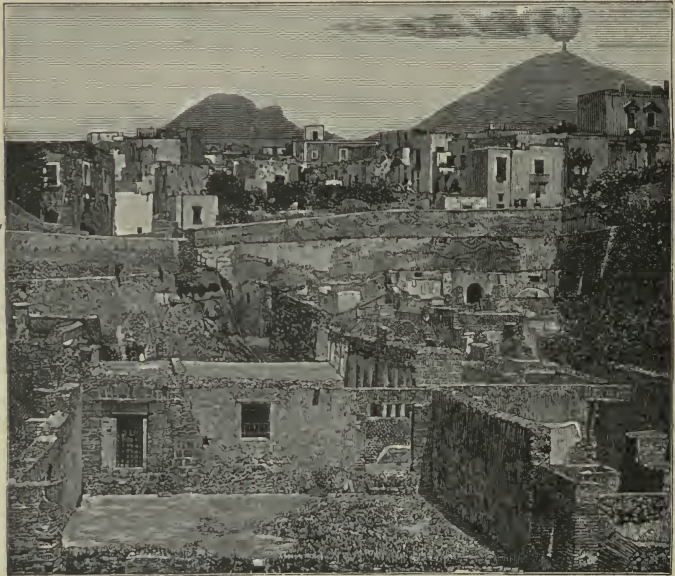
FIG. 111. Excavations in Herculaneum
